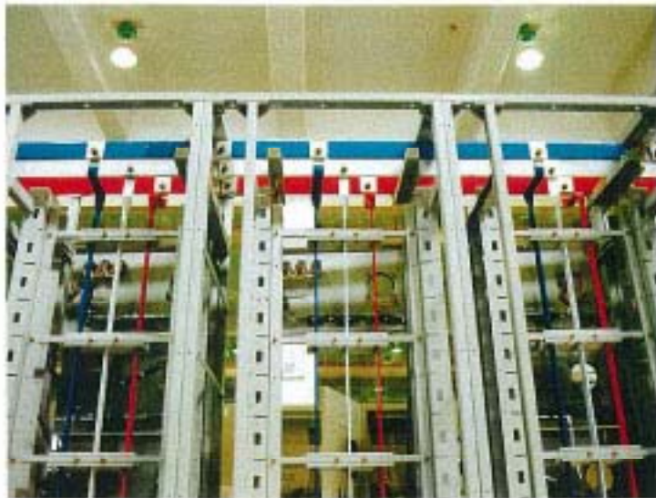
Fig.10 BUSBAR SYSTEM
