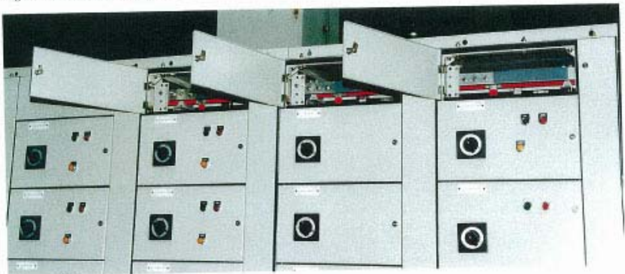
Fig.9 HORIZONTAL WIREWAY
