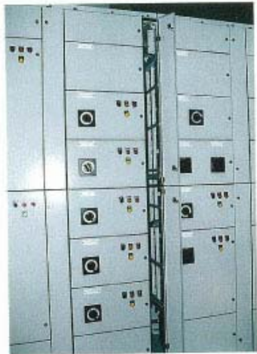
Fig.8 VERTICAL WIREWAY
